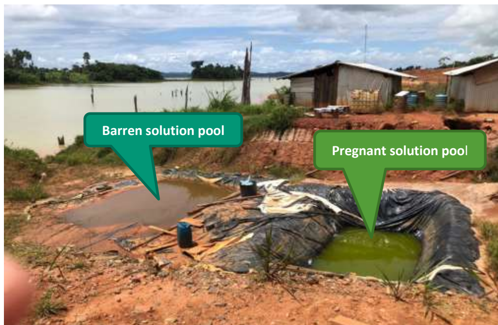
Figure 2. Pregnant and barren solution pools at Ero Bergi site
