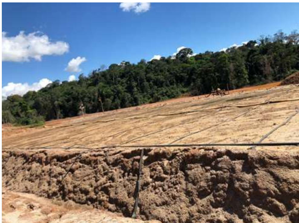
Figure 6. Heap leaching setup at Bohmila site
